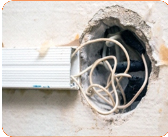
Fig 7.12 Be careful with exposed cables
