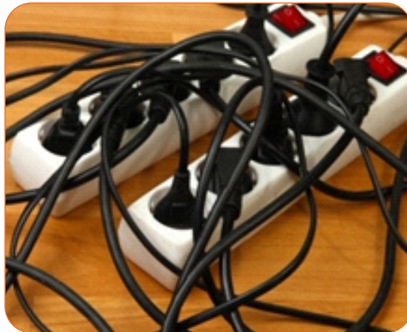
Fig 7.13 Overloaded extension cords
